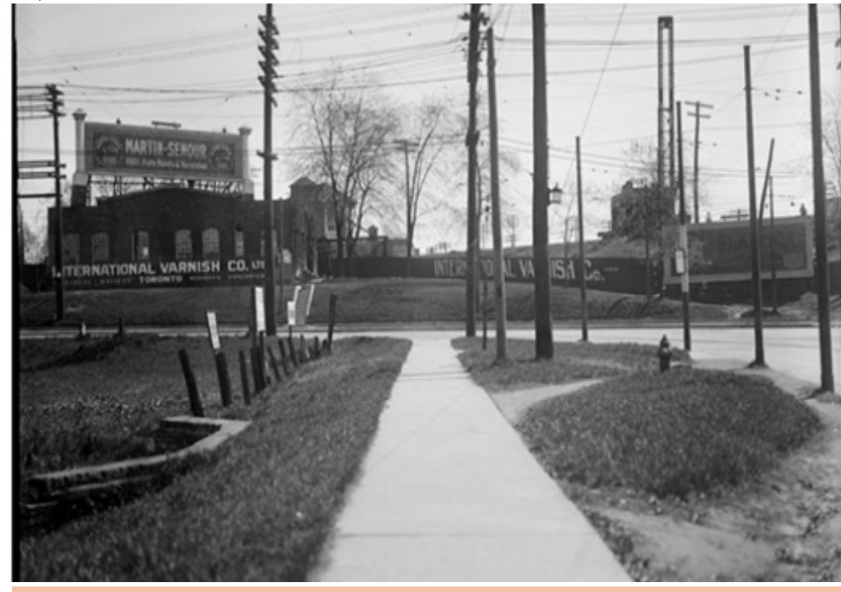
The International Varnish Co. complex which used to exist at the NE corner of Carlaw and Gerrard. Today the site serves as a No Frills supermarket.
